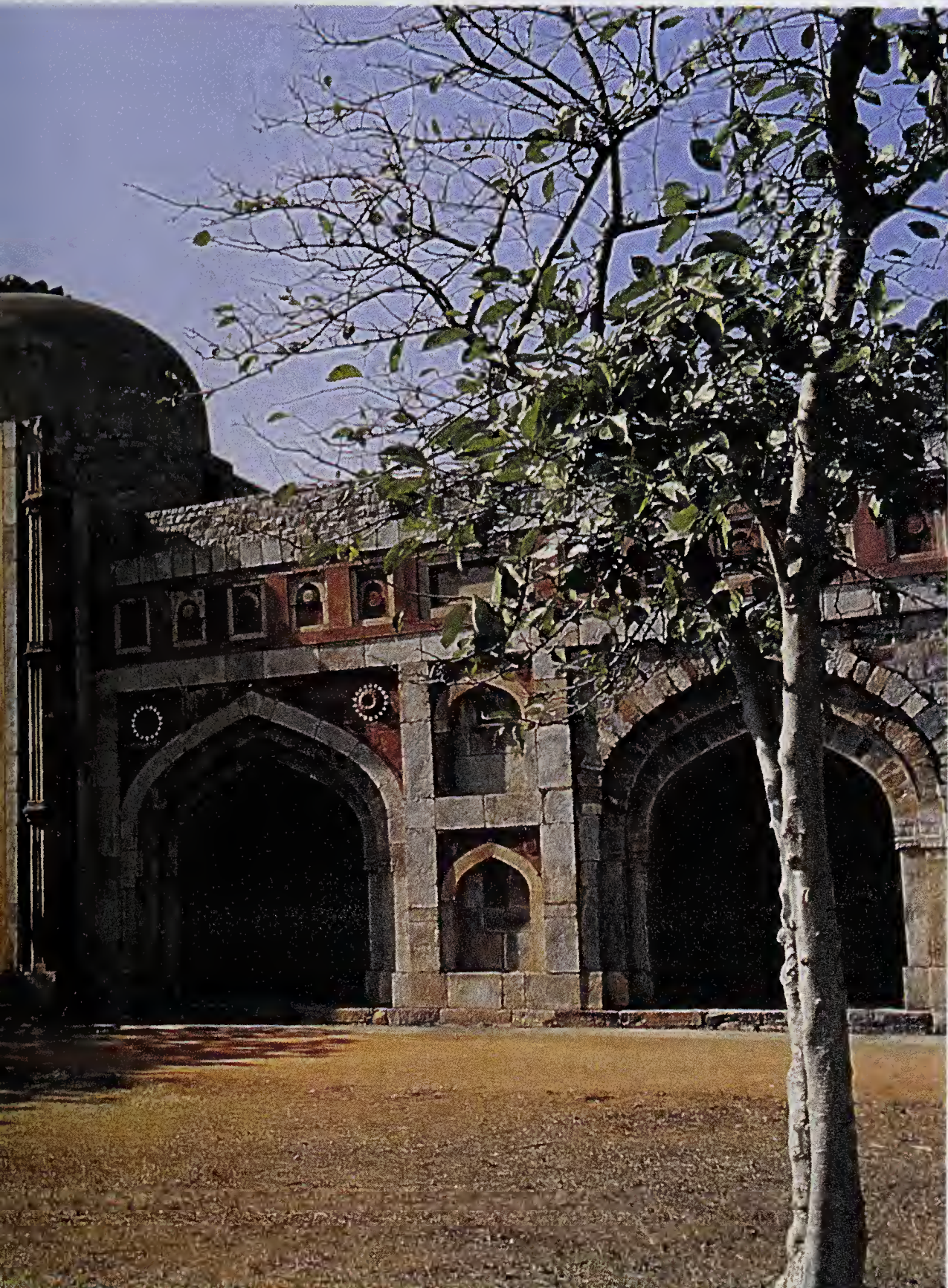
Above: Jamali-Kamali Mosque
